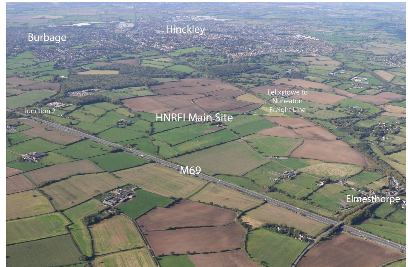
Fig.2 Aerial image of main HNRFI site with M69 in foreground looking towards Hinckley and Burbage.
