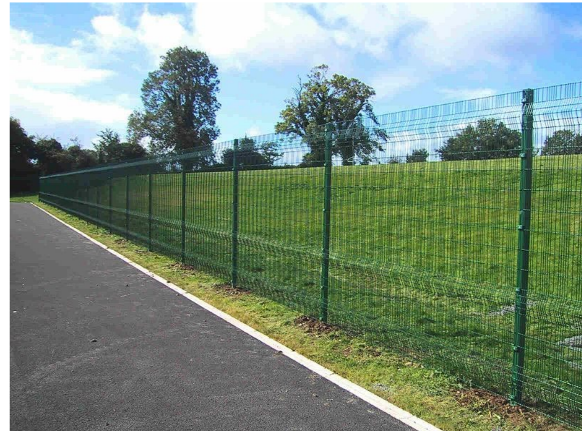
Fig 55. Typical boundary security fencing.
